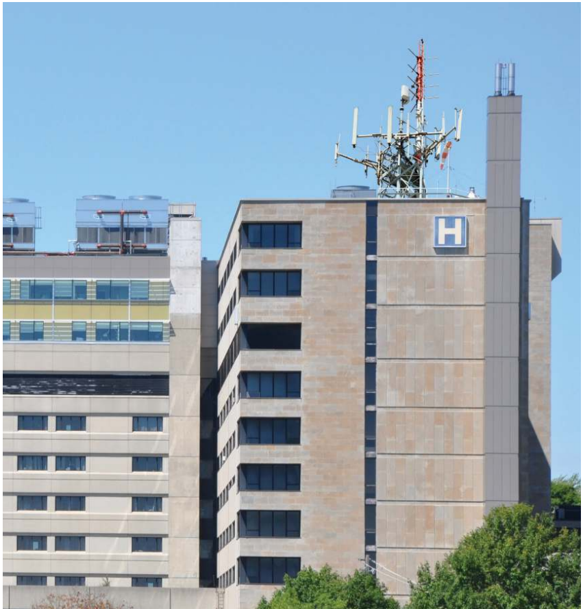
Figure 2. Antenna farm on roof of hospital
