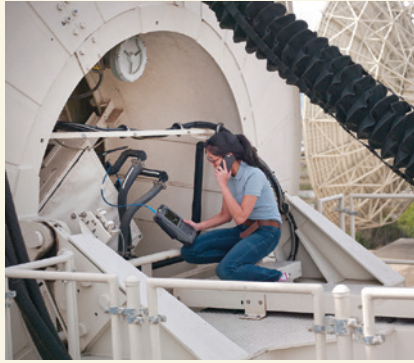
▲ Fig. 1 FieldFox handheld analyzers enable field personnel to fully characterize complex satellite earth stations with a single instrument. Photo courtesy of INTELSAT.
