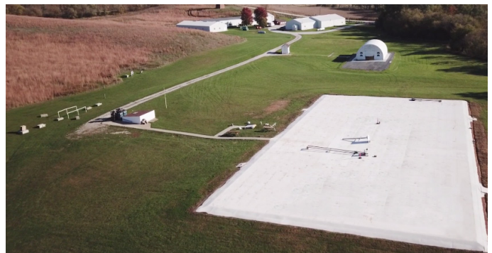
50x80 meter CALTS-compliant ground plane
